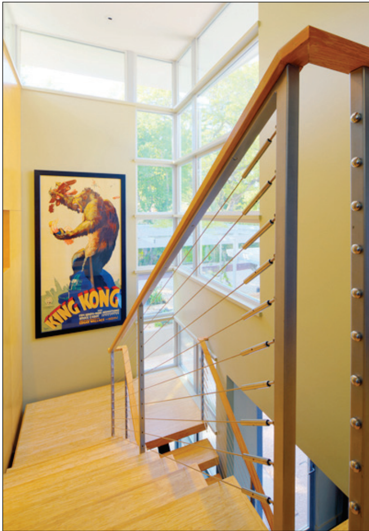
Interior stair railing with CableRail by Feeney Inc. Photo: Jonathan Jackson Photography
